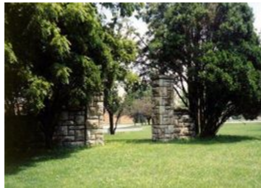
Below: Back gate.
