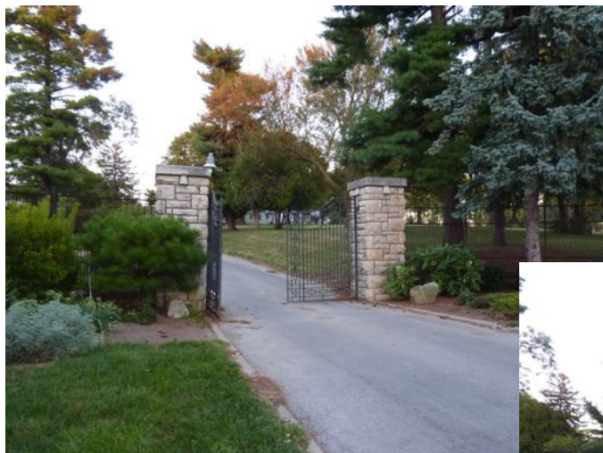
Front gate and fence.
